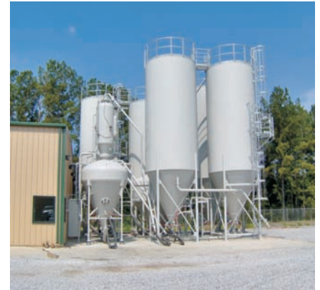
Vacuum/Pressure Plant Laurel, MS
